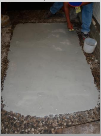
Makes surface harder, chemically more resistant, scratch resistant and capable of coping with heavy loads
