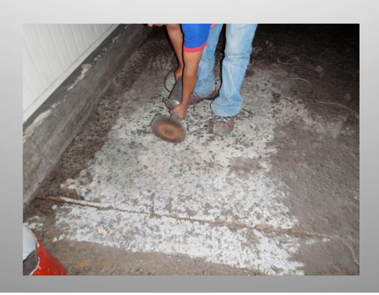
Chiseling the flooring is very labor intensive so we instead utilized mechanical tools to quickly prepare the surface taking out the loose concrete, damage screed, oil & grease, etc.
